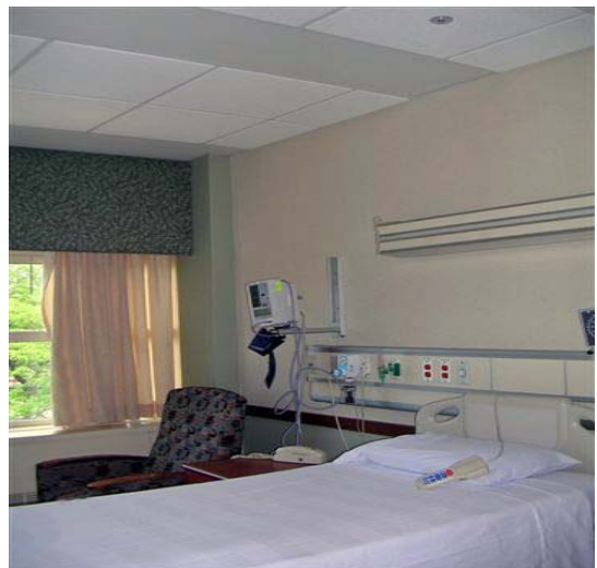
Patients experience a quiet environment because Mesurflo® valves eliminated pipe noise.
