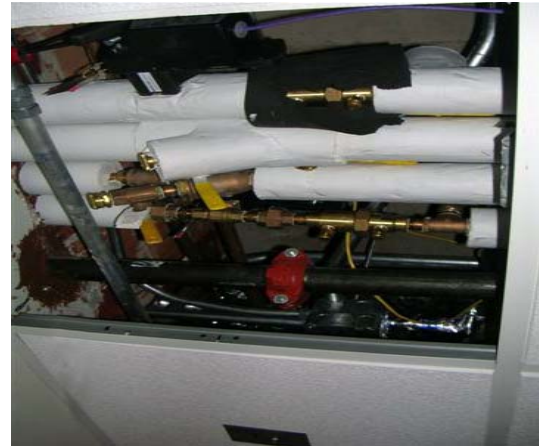
Mesurflo® valves eliminate the need to proportionally balance traditional manual balancing valves.
