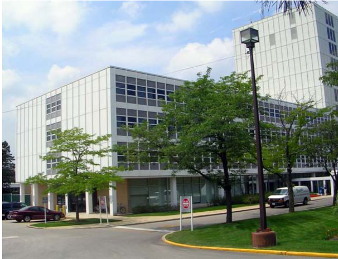
Northwest Community Hospital, Arlington Heights IL Phase 3 South Tower Patient Comfort Initiative
